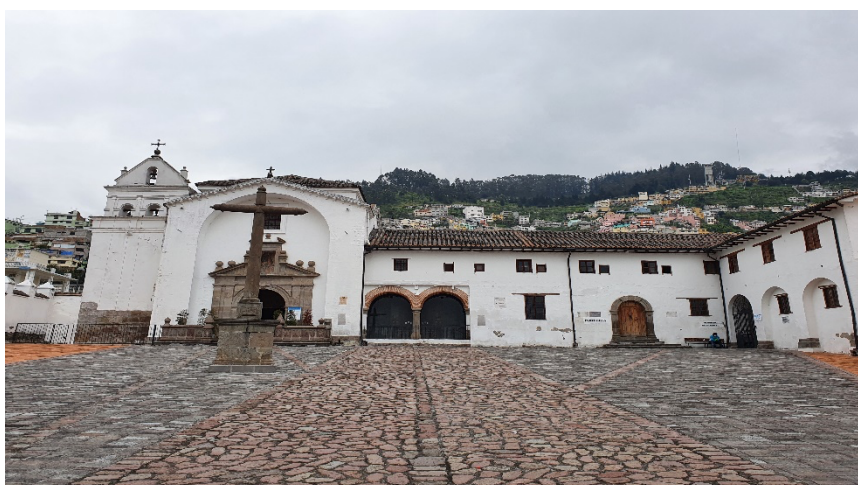
Figure 1. Main façade of the "San Diego" convent. Quito, Ecuador
